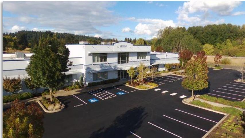
Delta Computer System’s headquarters in Battle Ground, WA
